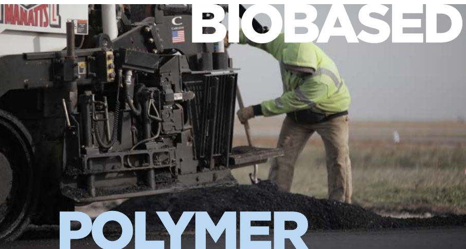
A new biobased polymer for asphalt made from high oleic soybean oil offers a lower-cost and cleaner alternative to the traditional binding agents used in asphalt. Photo Credit: United Soybean Board
